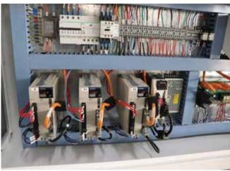
"Precision rack and pinion drive system and low-profile drive system allowing for easy loading from any side. Internal electrical cabinet featuring yaskawa motor drivers, and the automatic focus-sing Raytool laser head.
